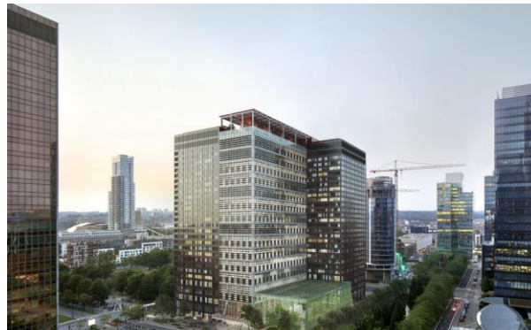
ZIN – OFFICES 100% PRELET 110,000 M 2 | BRUSSELS NORTH AREA
